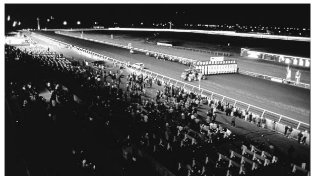
Figure 1. This racetrack is lit by clustered banks on individual structural towers to provide the lighting needs of both contestants and a large number of spectators.
